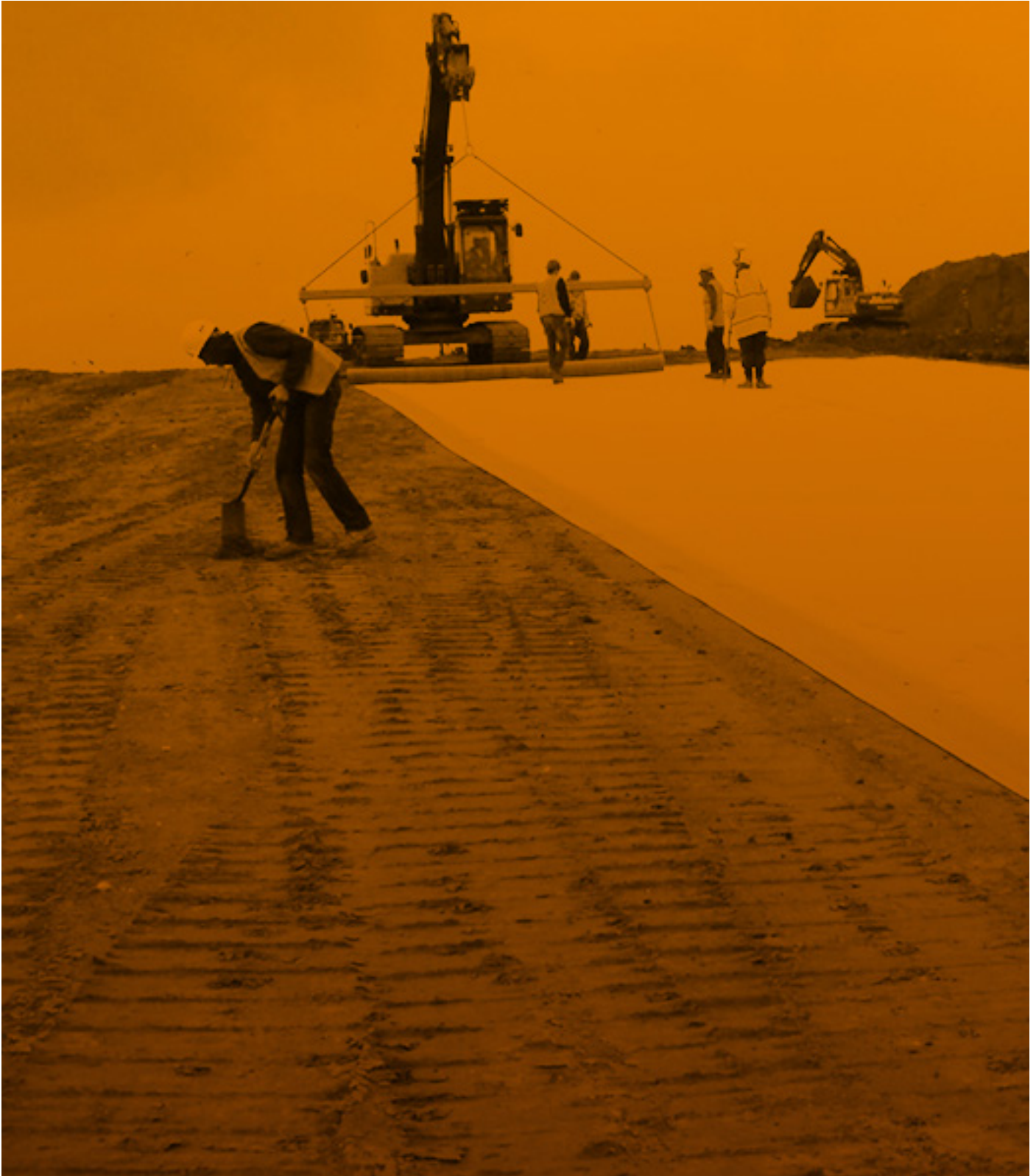
PREPARATION FOR PLACING SOIL COVER
